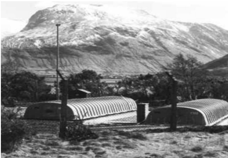
Rys. 5. Oczyszczalnia z TZB – Corpach, Anglia Fig. 5. The wastewater treatment plant RBC – Corpach, United Kingdom
